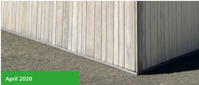
CLADDING PROJECT, NORTH AMERICA
