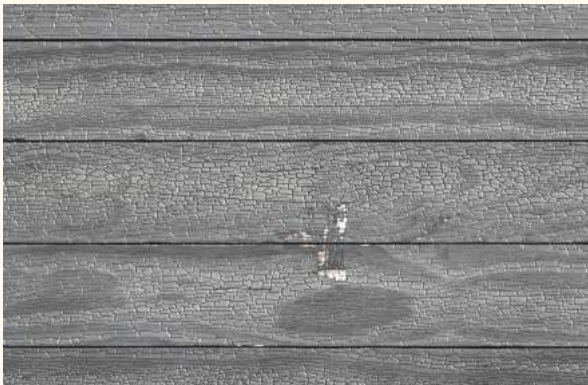
Damage from a ladder - scraped SSB Gator®
