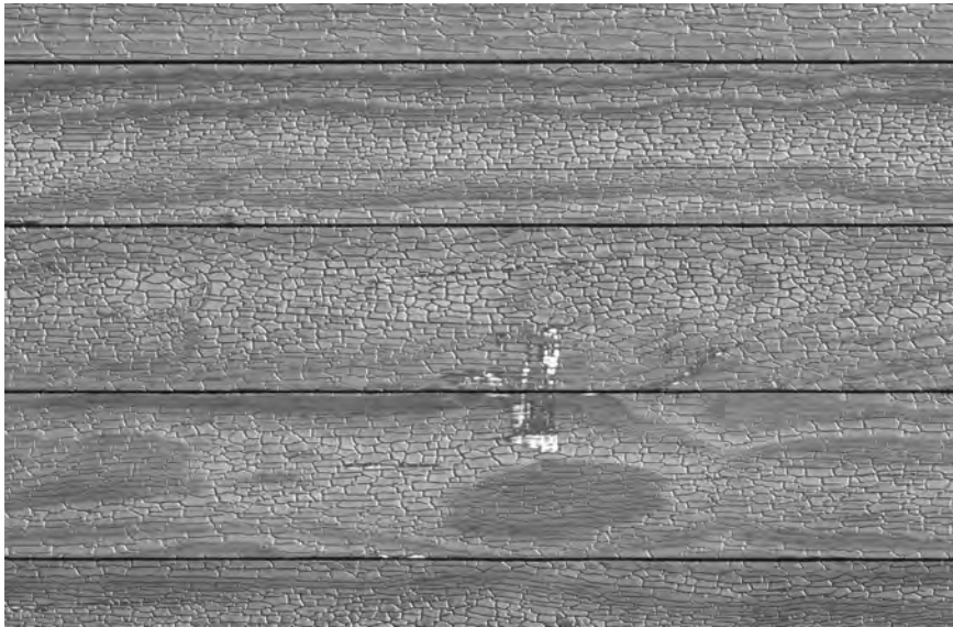
Damage from a ladder - scraped SSB Gator™
